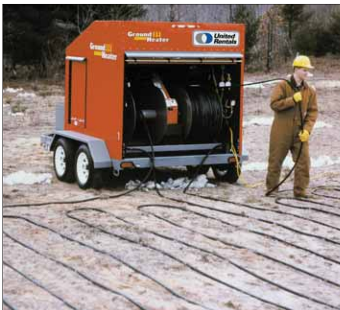
A ground heater will thaw frozen ground or pre-heat concrete forms to keep construction moving during cold winter months.
